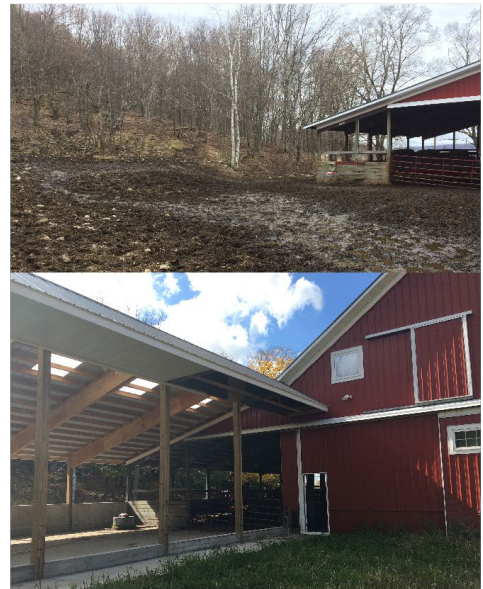
Heavy use area before ( top ) and after ( bottom ) implementation of a heavy use area protection BMP. This project reduced erosion and surface runoff of agricultural waste.
